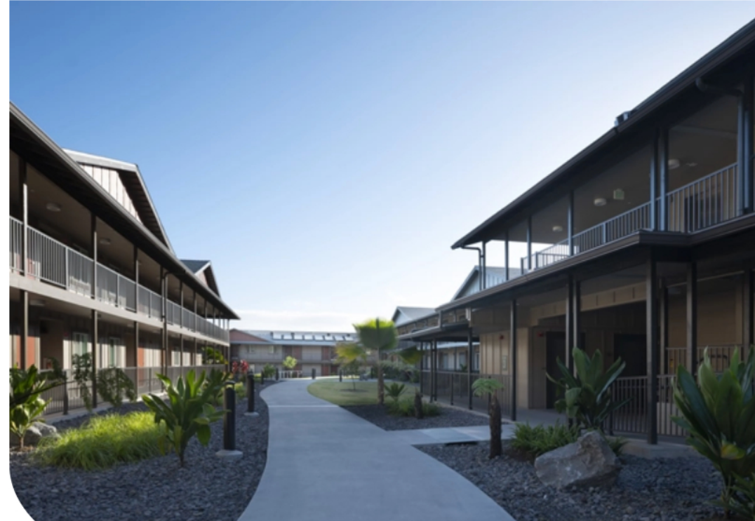
Hale Nā Koa 'O Hanakahi, which roughly translates to "House of the Warrior," is Hawai'i's first income-restricted rental community targeting senior veterans and their surviving spouses. Photo credit: EAH Housing
